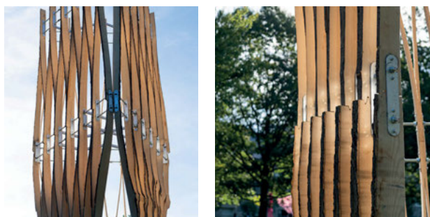
Fig. 10: Left: connection between panels C and D; Right: splice connection. (Photos by Cynthia Kuo)
