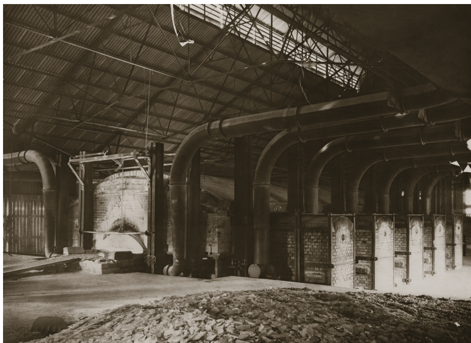
2 Tank furnace, late 19th or early 20th century, Belgium, photographer unknown.
