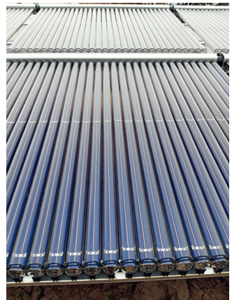
Figure 14.2: Schematic diagram of vacuum tubes with strip absorber and cylindrical absorber (left) (source: target GmbH [Geiger]), photo of a vacuum tube collector (right).
