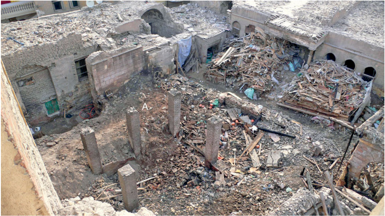
Fig. 1: The courtyard of an abandoned ‘palace’ in the Darb el-Ahmar district of Cairo. ‘A’ is the centre of underground combustion, marked by orange-coloured earth and blackening of an adjacent wall. The combustion spread throughout the debris, eventually causing architectural woodwork at the back of the building (right-hand edge of the picture) to catch fire.
