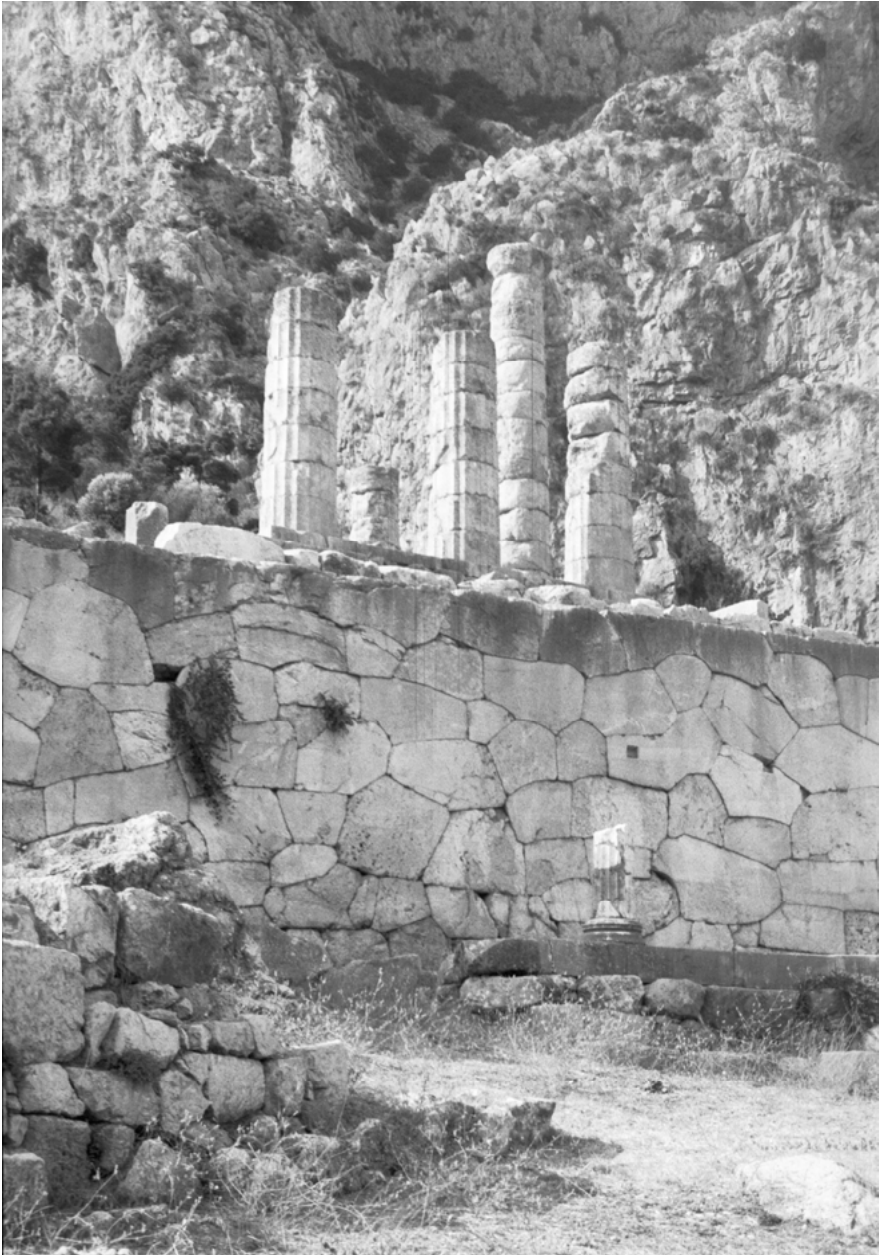
Fig. 1: Delphi, polygonal wall and the temple of Apollo; < https://commons.wikimedia.org/wiki/File:Supporting_polygonal_masonry_of_Temple_of_Apollo,_Delphi,_Dlfi301.jpg > (accessed on 19 April 2021). CC-BY-SA-4.0.
