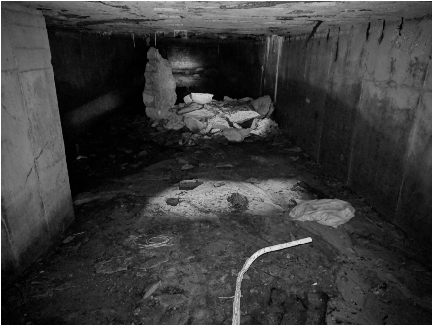
Figure 6.2: Underground tunnel with gravel from collapsed ceiling.
