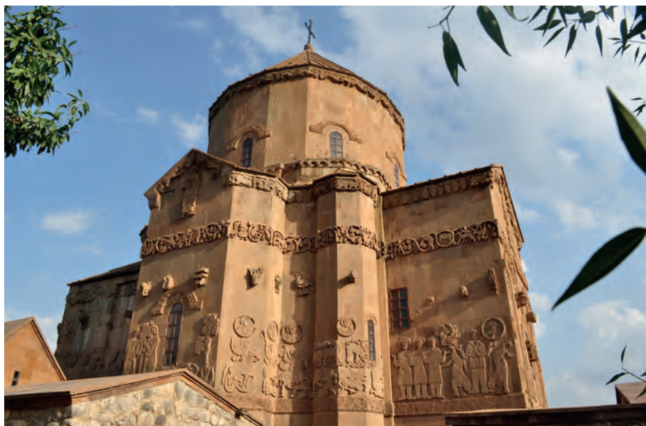
Fig. 6: Church of the Holy Cross, Lake Van, Turkey, photo by Gorčin Dizdar
