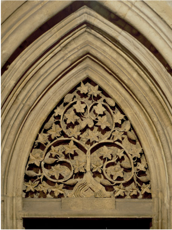
Fig. 4: Prague Altneuschul, c. 1280, entrance tympanon. Photograph: author.
