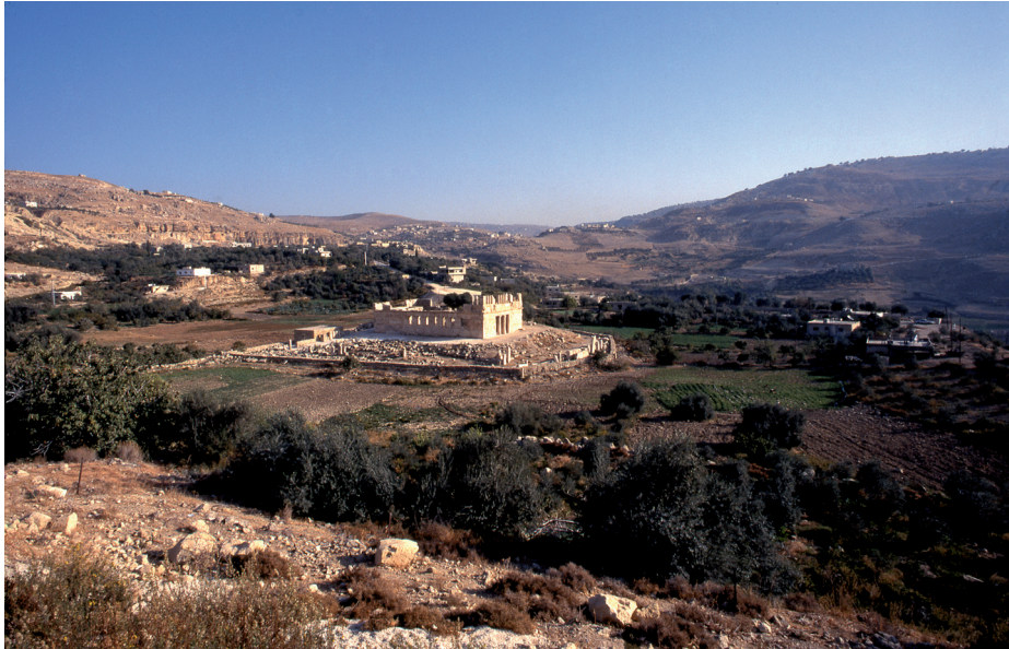
Fig. 17. The Tobiad fortress , a possible location of the “pools in Hesbon” (Song 7:5). Palace building of c. 200–175 BCE in front of the tell of Tur ‘Abid/Qasr al-‘Abd (Jordan). Photographer Garo Nalbandian.
