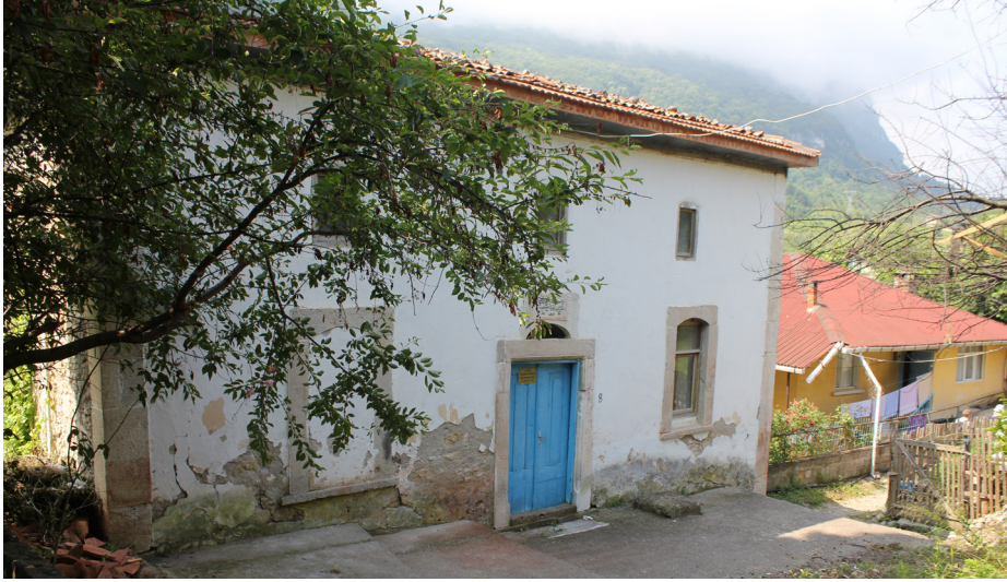
Fig. 14.24: Stone-built architecture at Gideros East. (CAP-P2/1799).
