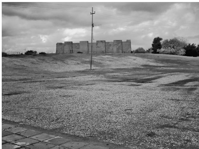
Fig. 24 | Leveling of the area south of the Temple of Ninmakh (State Board of Antiquities and Heritage, Iraq).
