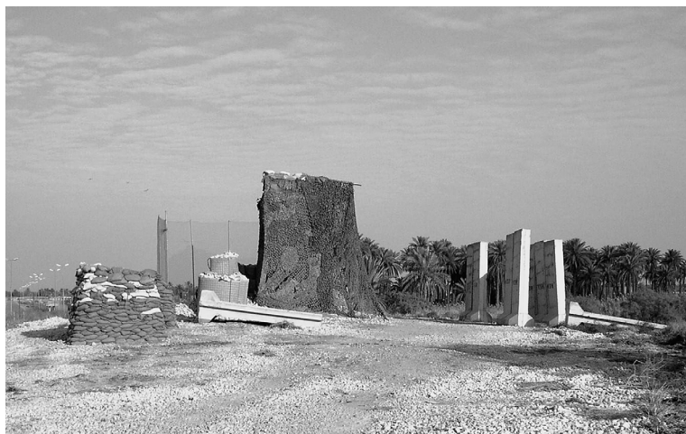
Fig. 13 | Sandbags, HESCO containers and concrete T-walls at Babylon (J. E. Curtis).
