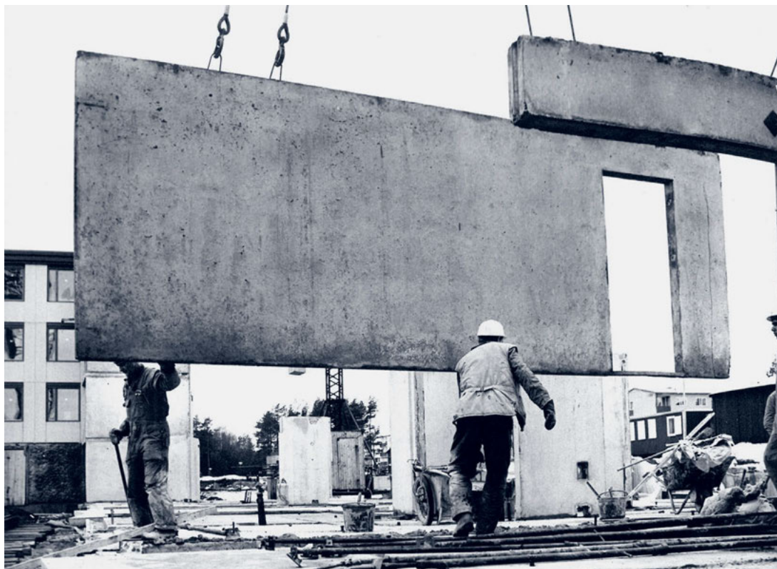
The construction site of the project Kv. Söderby, built by Ohlsson & Skarne using the Heavyweight System.
