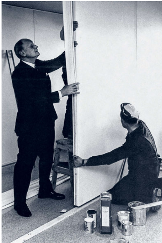
Allan Skarne assisting in the mounting of a prefabricated interior wall element in the project Kv. Diset in Uppsala, the prototype for the S66 System.
