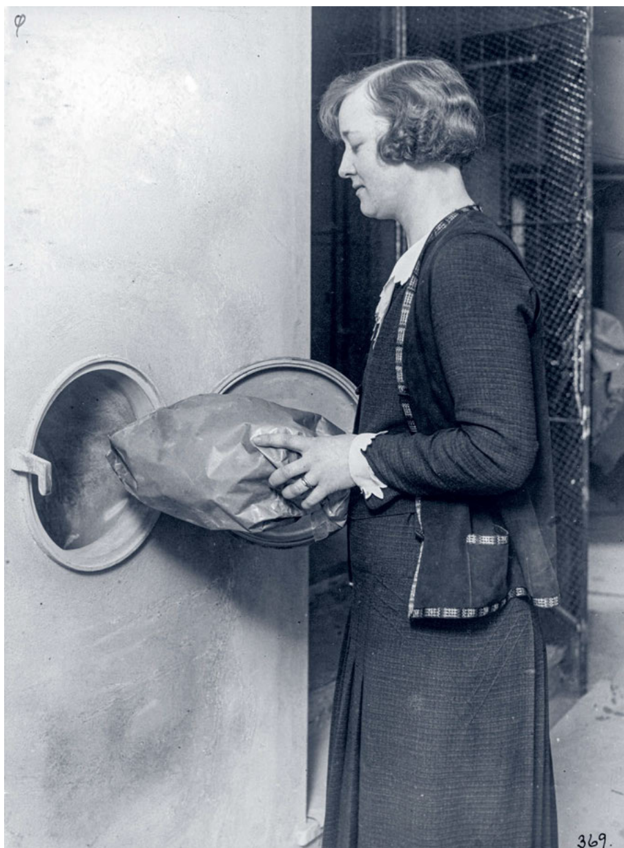
HSB was first to develop this kind of garbage disposal on every floor of their mass housing estates from 1928 and onwards. Sven Wallander received a Swedish patent for the garbage chute in 1934. Catherine Bauer collected the photograph of the garbage chute in her personal research archive on housing in Sweden.
