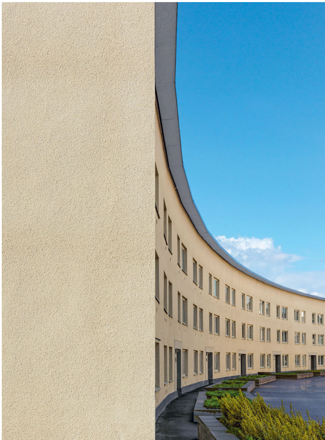
Navestad's original ornamental concrete panels and balcony fronts were replaced in 2003 with a smooth plaster façade in various colors. Photographed by John Håkansson in 2023.
