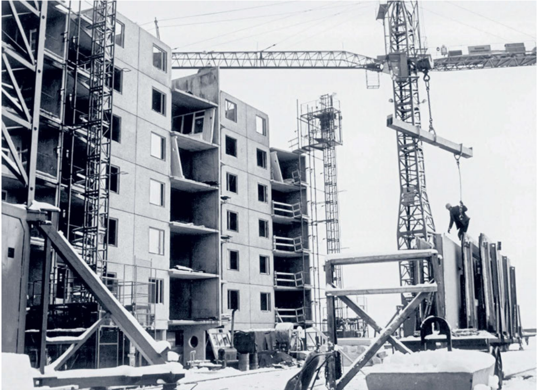
Navestad's housing estate under construction in the winter of 1969. The new industrial building methods that Erik Ahlin and Arne Johansson developed for Norrköpings panel fabrik allowed for construction during the winter. Note the snow on the concrete panels and building cranes.
