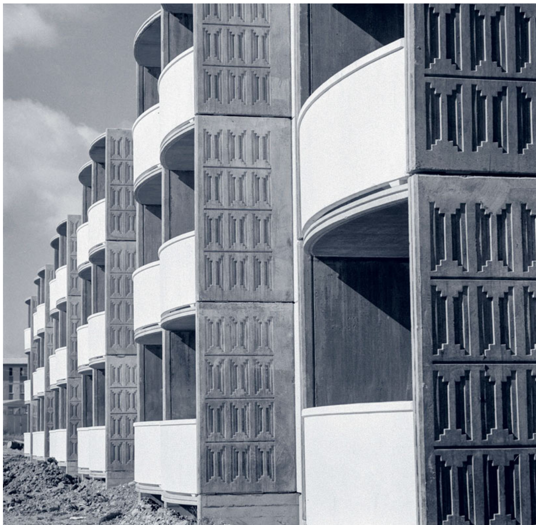
Designed by Erik Ahlin, this housing estate in Norrköping was the first to be built in prefabricated concrete panels, delivered by Norrköpings Panelfabrik. The panels had a relief pattern by the silversmith Sigurd Persson and curved concrete balconies. Photograph by Sune Sundahl for the magazine Betongindustrin , 1964.
