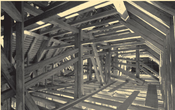
▲ Fig. 5 | Abb. 5: With the hanging truss roof structure he built from 1764 to 1767 in a church in Wädenswil (Switzerland), Hans Ulrich Grubenmann succeeded in keeping the 21 meters by 36 meters oratory free of columns.
