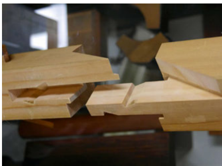
◀▼ Fig. 2 | Abb. 2: Examples from the collection of wood joints of Shimizu Corporation furniture carpentry, Tokyo. Photos © Karin Raith
