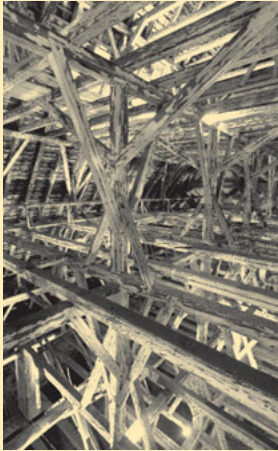
▲ Fig. 4 | Abb. 4: The five-story Gothic roof truss built by Thomas Schweinebacher from 1503 to 1518 in Schwaz (Austria).
