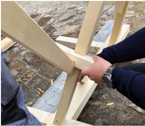
▲ Fig. 7a | Abb. 7a: Locking of two vertical criss-crossing members by a third horizontal part inserted from above.
