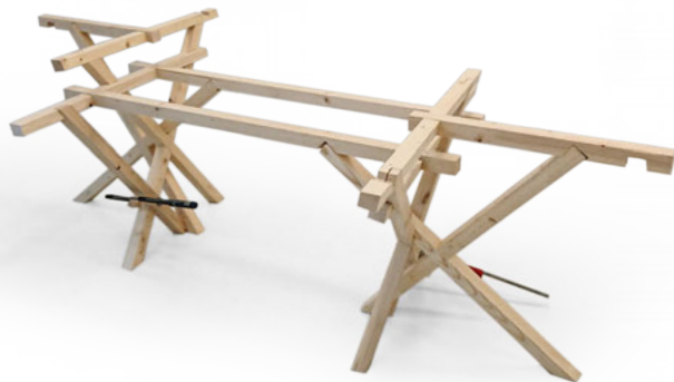
▲ Fig. 8 | Abb. 8: The splitting of otherwise continuous beams at the top horizontal layer affected a high density of notches where the tabletop splits. As a result, some connections had to be screwed for fixation, furthermore the tabletop panel had to be screwed.
