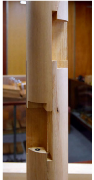
◀▼ Fig. 2 | Abb. 2: Examples from the collection of wood joints of Shimizu Corporation furniture carpentry, Tokyo. Photos © Karin Raith
