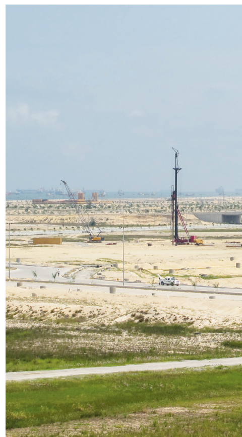
Land reclamation and luxury towers under construction. Eko Atlantic, 2018
