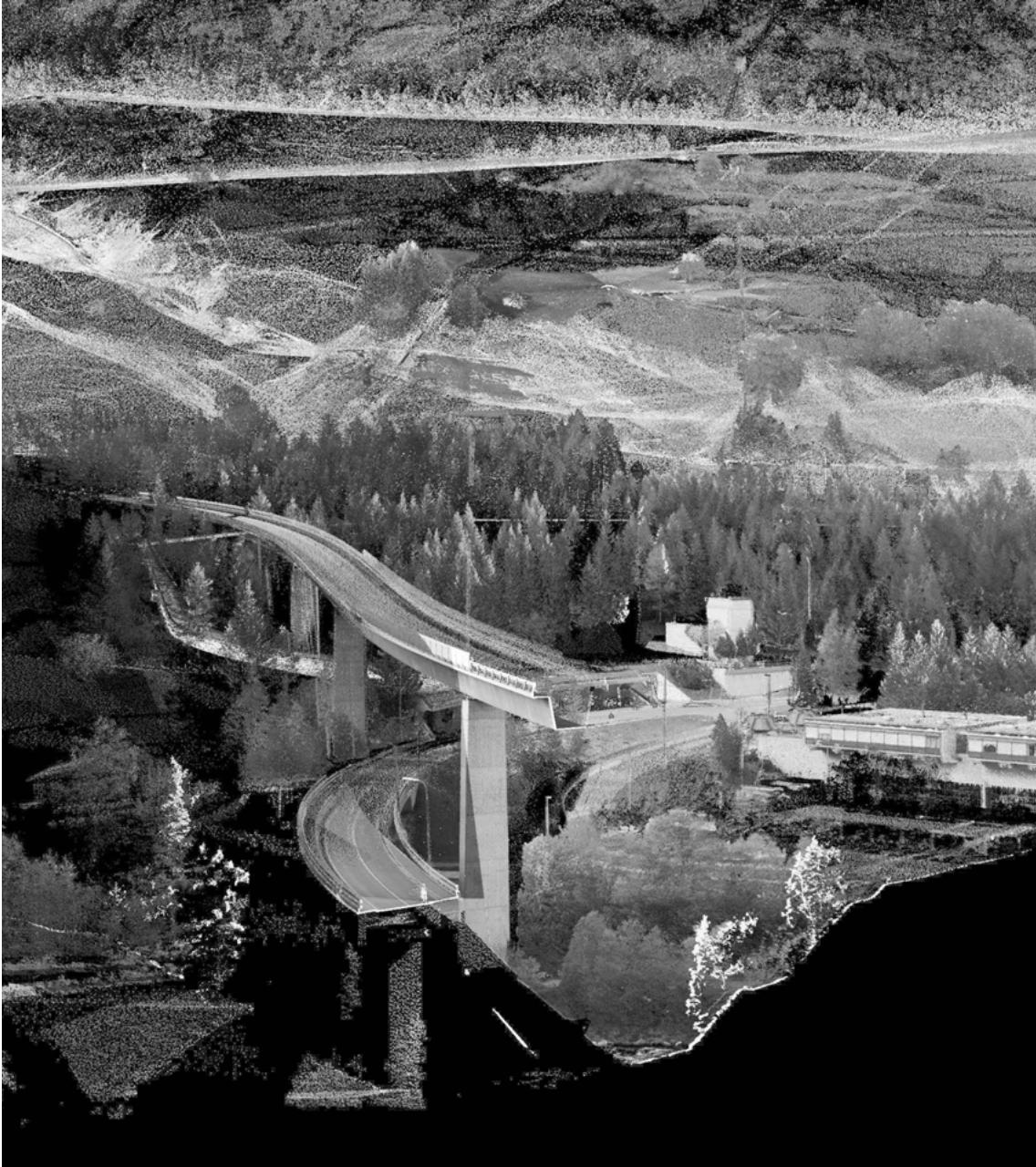
Fig. 2 (p. 100) Section on the old Tremola Road in Ticino Switzerland with the Gotthard Motorway tunnel below, 2014
