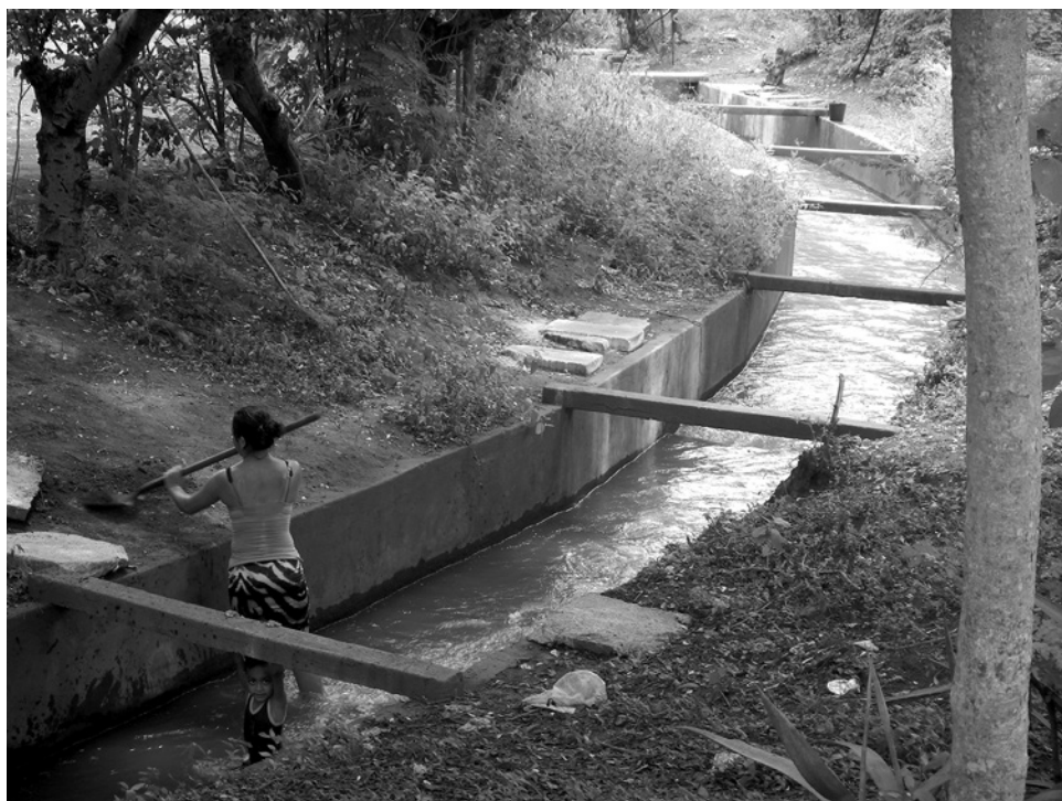
FIGURE 3.1 Maintaining the embankment on an irrigation canal. Photo by the author.
