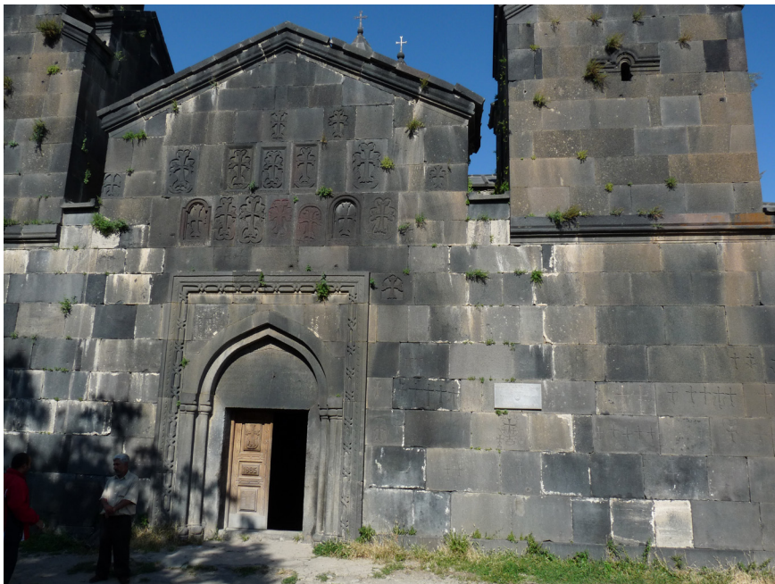
FIGURE 20. The entrance to the gavit at Teler Vank'. The endowment inscription is located in the arched lintel above the door. Photo by the author.
