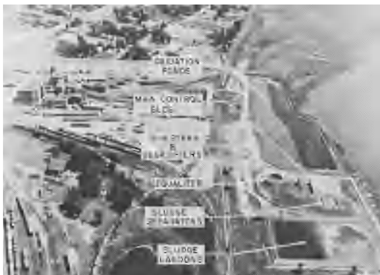
Figure 2. Full scale anaerobic contact waste treatment plant, Wilson & Co. Inc., Albert Lea, Minnesota USA
